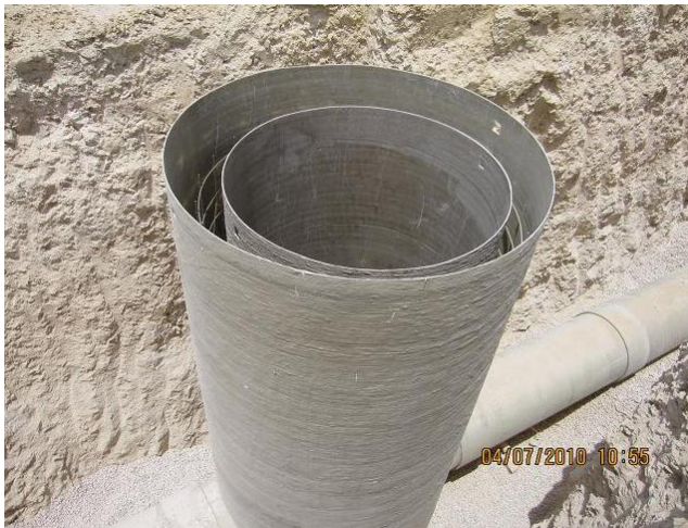
Figure 4: Liner Manhole
